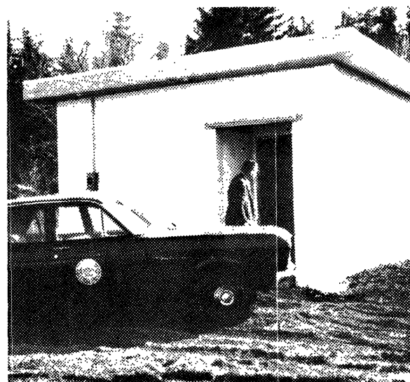
The Beaver Central Office Building houses the new automatic switching equipment and carrier facilities. The building located next to Loushin's Richfield was constructed by local contractor Don Quick. Electrical work was sub-contracted to Fletcher Electric of Forks.
